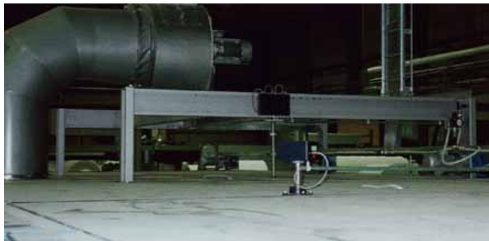
Typical installation: thermoset OMT/VMT between two circulating-air ducts
