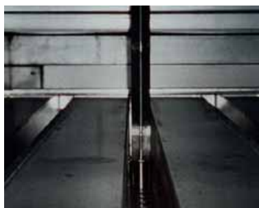
Typical installation: thermoset OMT/VMT between two circulating-air ducts
