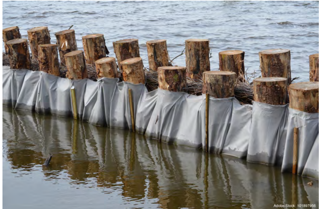
Fig. 3: Flood protection can only fulfil its task with the right coating.
